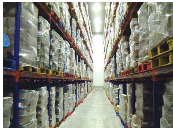
Lights - 132W HB2 Illumination at floor level - 420 lux
